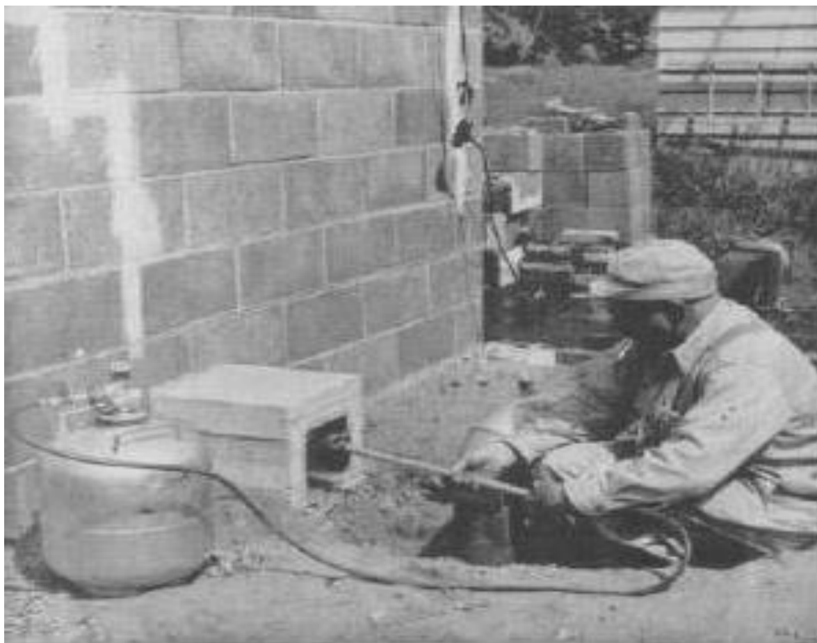
Igniting the kiln charge with a torch.
